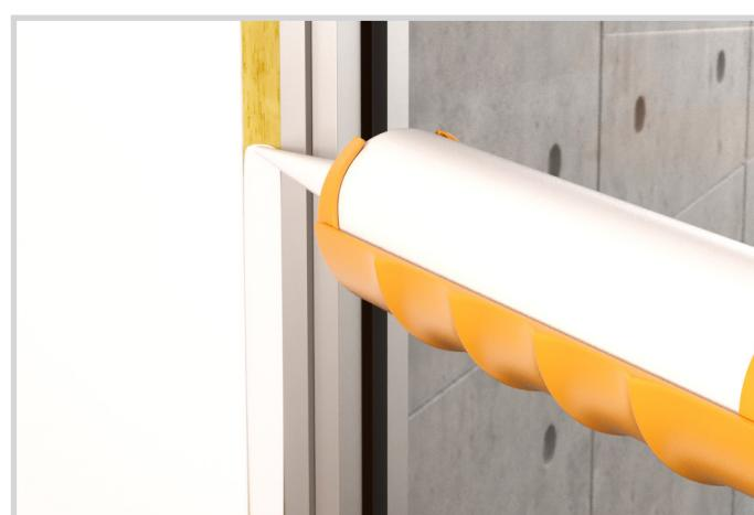
7.3 - use silicone caulk to seal the area between the structure and frame.
